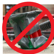
Angled Edges Help Prevent Damage Caused by Rebar
